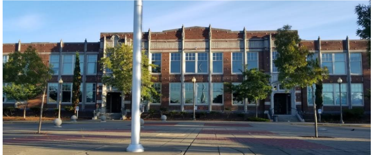
Hilltop Heritage Middle School, Installed 2021
